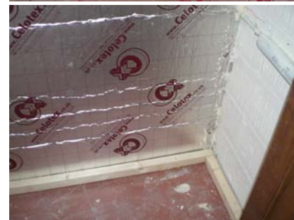
Photos: Solid wall and floor insulation Mar 09
