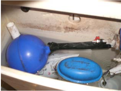
Photos: Toilet hippos installed in the cisterns
